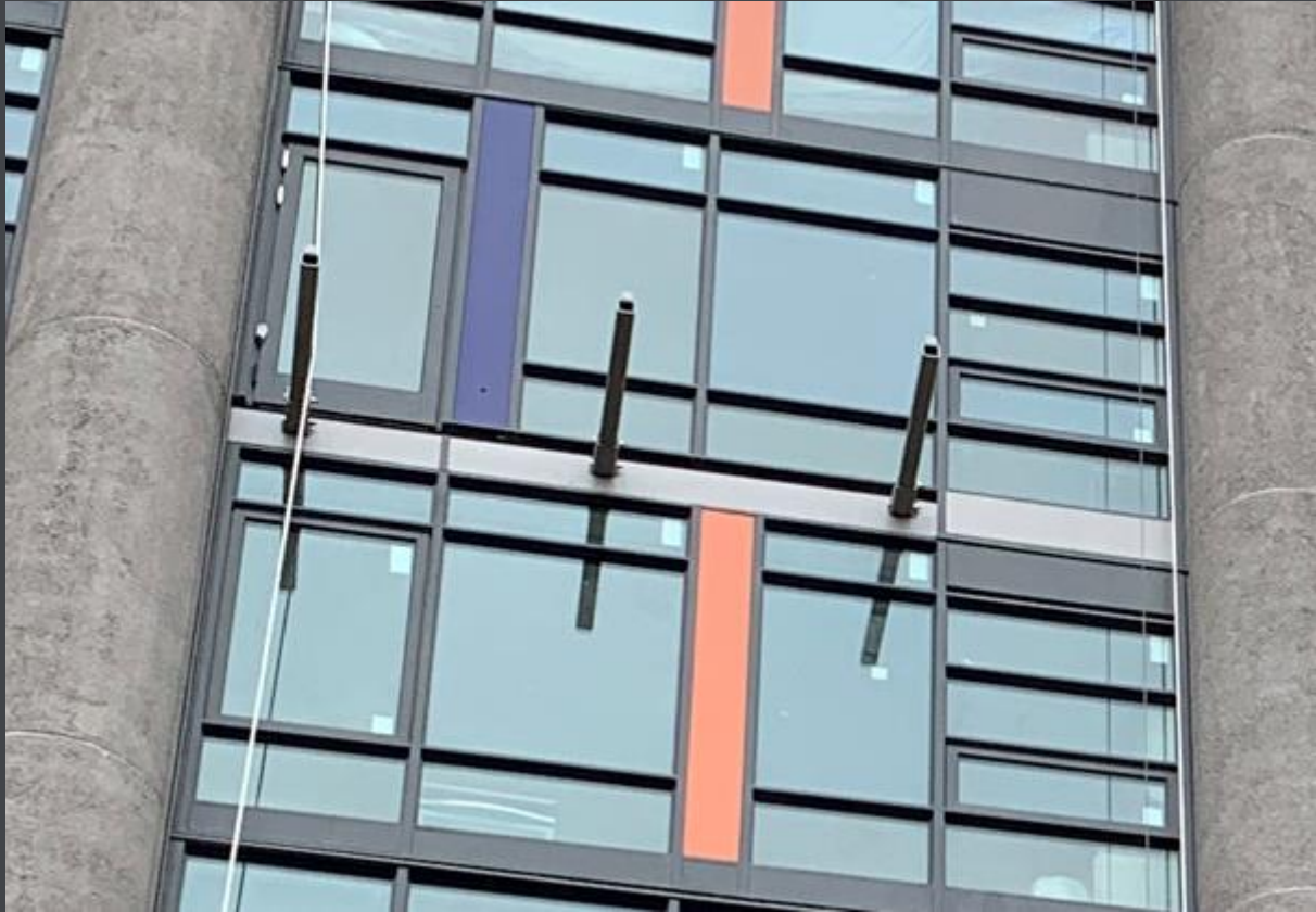
Installation of Outriggers for Balconies
