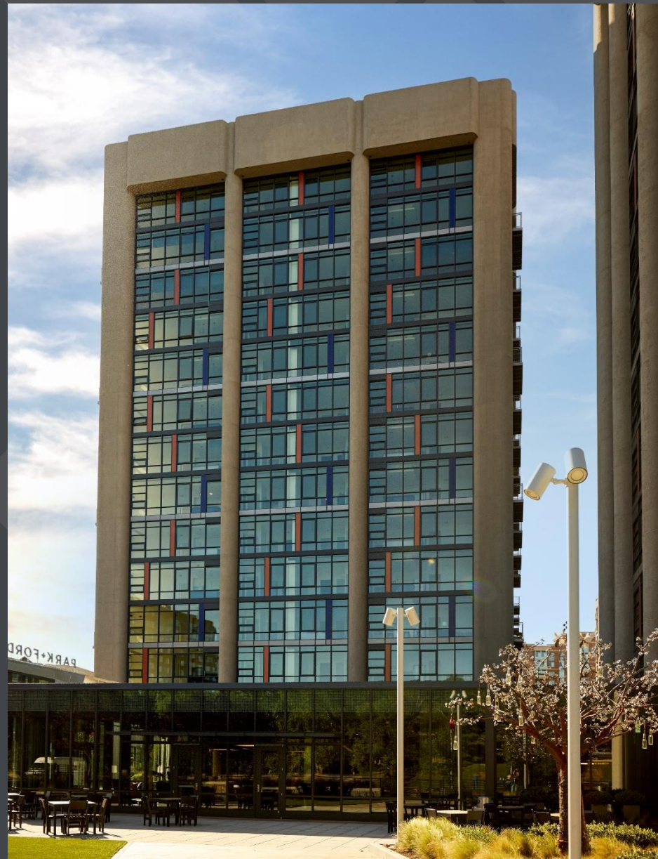
FORD BUILDING AND LINK LOBBY
