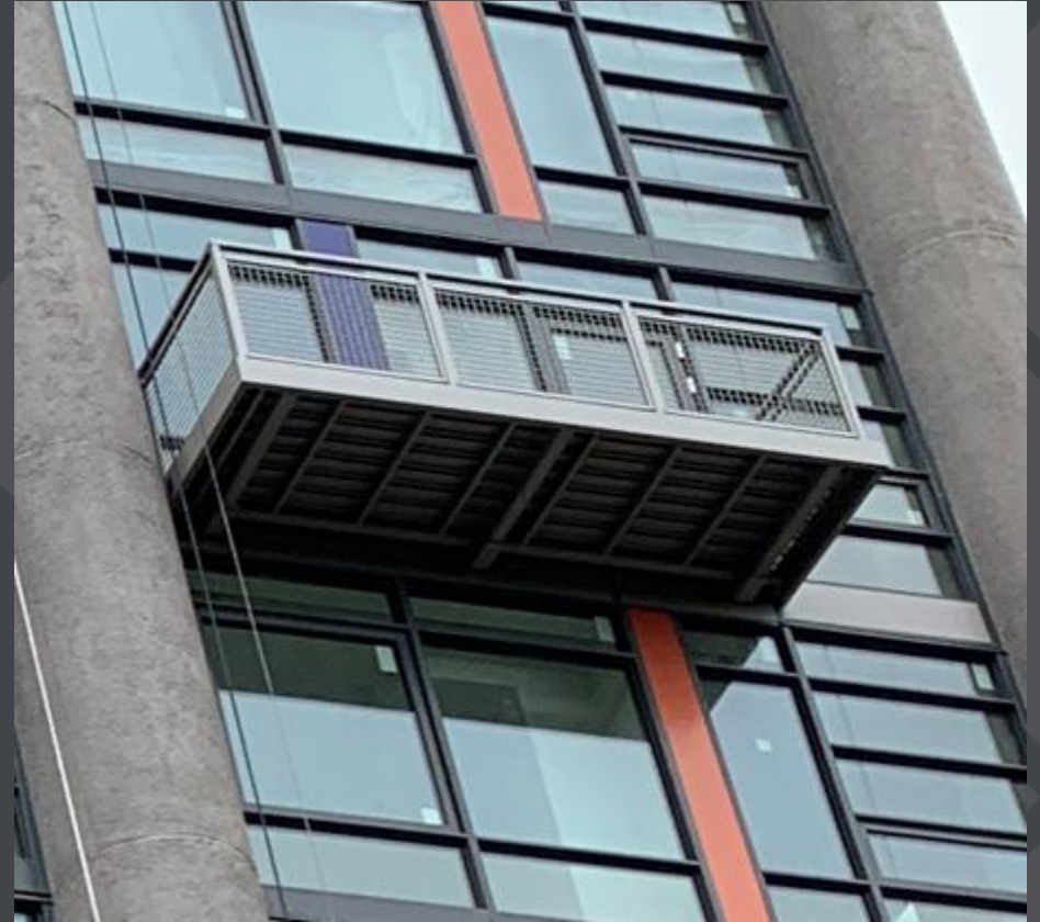
Balconies Set in Place from Top of Building to Bottom
