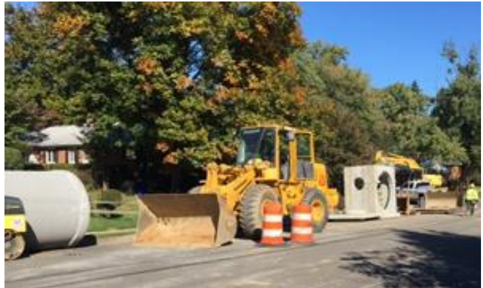
West Little Pimmit Run, under construction 24 th and Rockingham, under construction
