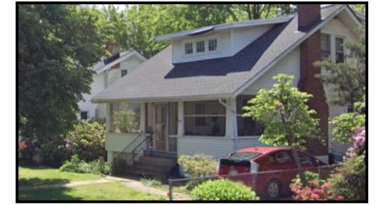
Typical Aurora Highlands House on 23 rd Street, ~25' tall
